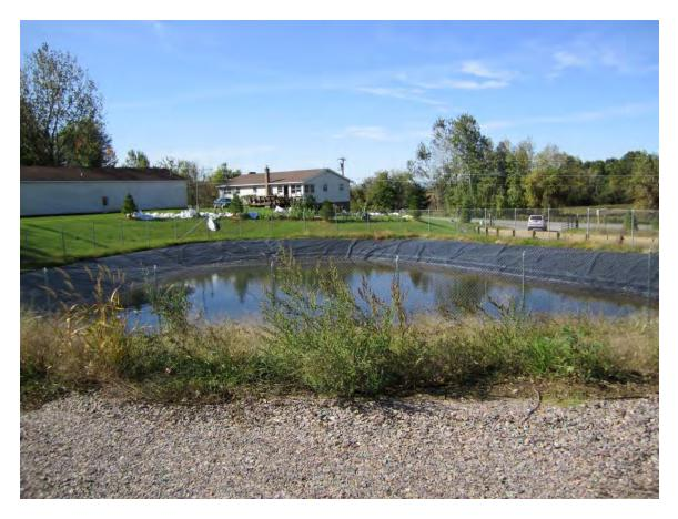
*Figure 8: Lined pond for collecting leachates (and rain water) during active phase 2 composting. The water in this pond is almost free of contamination. The residence on the other side of the pond labeled L in figure 1 is owned by CSWD and is rented at a reduced rate.*
