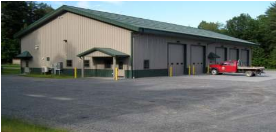
The new Department of Public Works garage on North Road.
